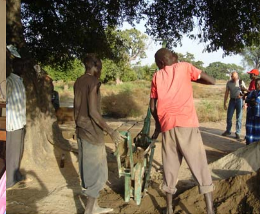
Masonry project run by Save the Children/Sweden in Malual Kon.
