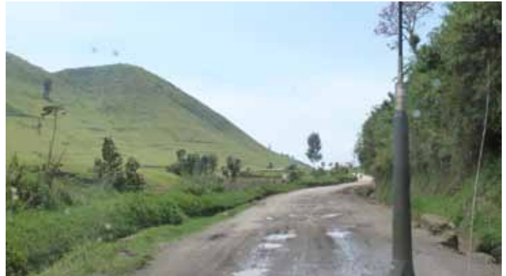
The road from Goma to Burora, North Kivu, DRC. © Nadia Tabaro/WRC.
