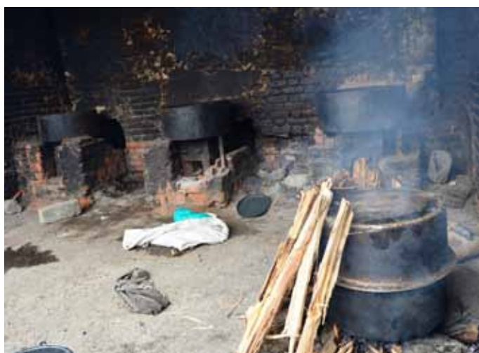
In the back, improved stoves constructed by Mercy Corps in the prison of Muzenze in 2011. In the front, a traditional stove in use. © Alvaro Trincado
